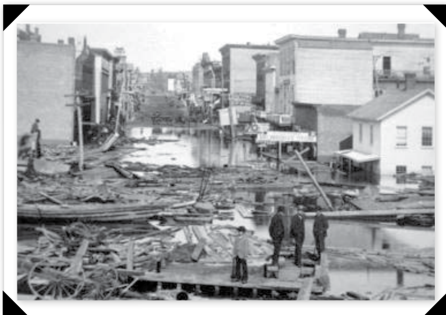
1941 Flood — Chippewa River.
